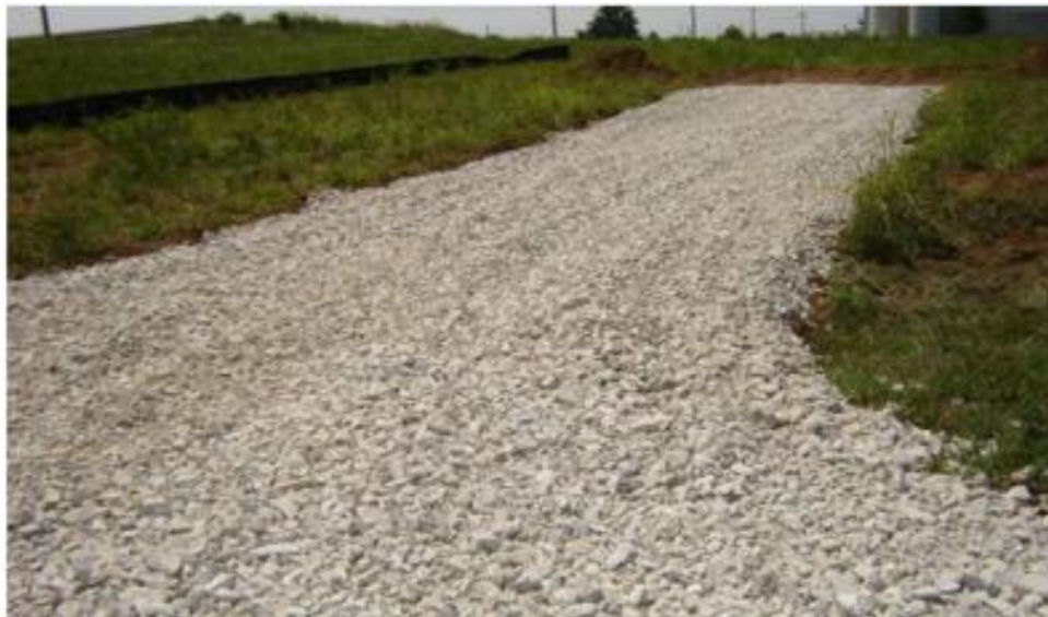
Plate 7: Temporary access track
